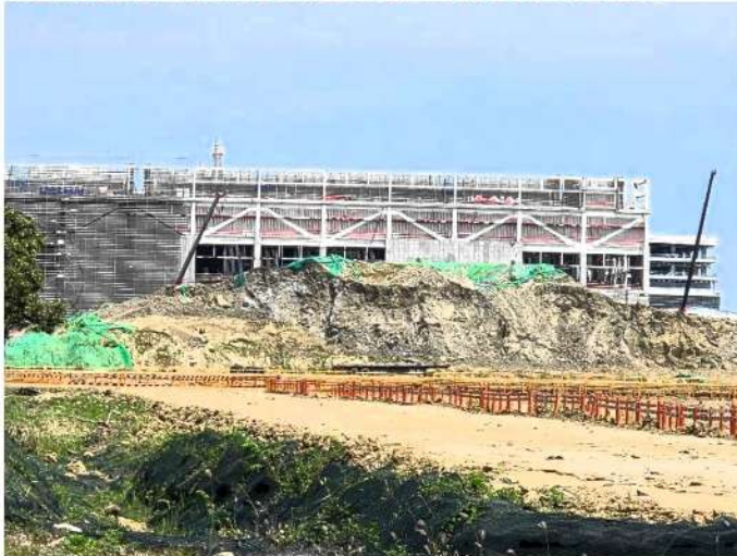
FIGURE 12A: AP7P2 FAB'S SHELL IS ABOUT TO BE COMPLETED
