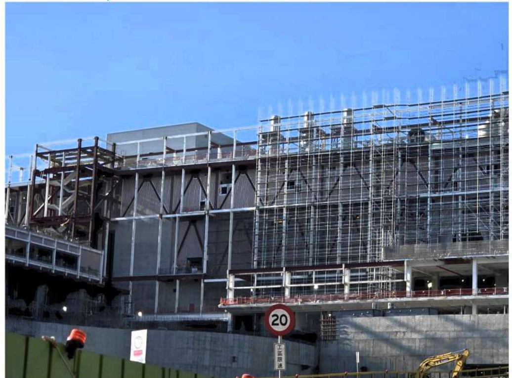
FIGURE 10: FAB22 P3/4: LOOKS THE FASTEST AMONG ALL IN-CONSTRUCTION NEW FABs
