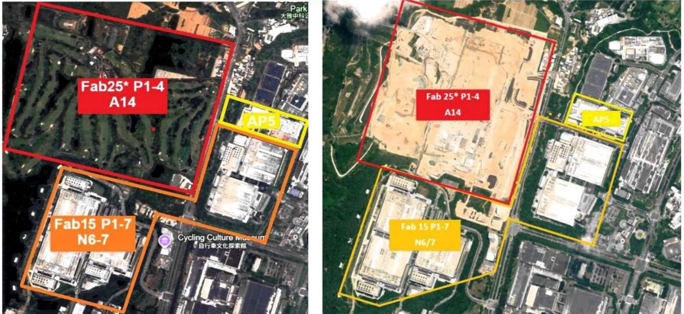
FIGURE 7: TSMC'S FAB CAMPUS IN TAICHUNG (CENTRAL TAIWAN) AND THE CONSTRUCTION PROGRESS COMPARISON (2025 VS NOW)
